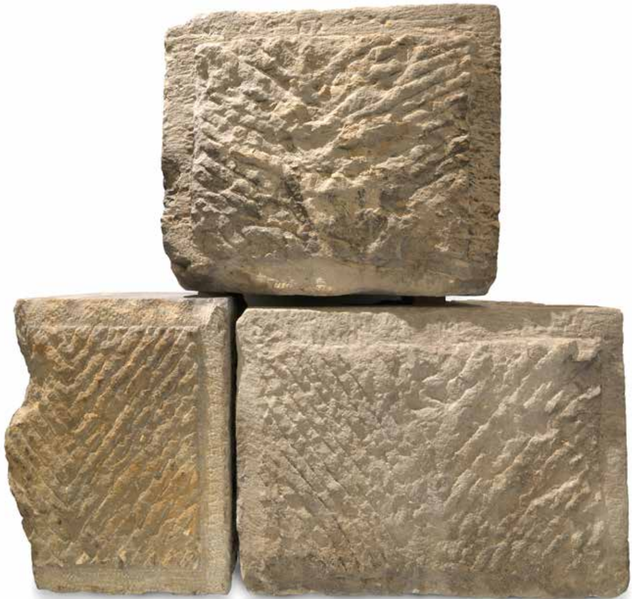
Fig. 5 - Facing ashlar from the fortification wall of the legionary fortress of Vindobona
