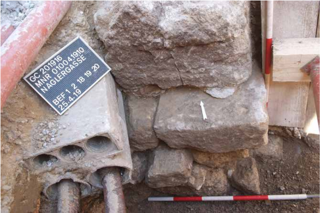
Fig. 6 - Ashlar, stone base and foundation on the western side of the porta decumana gateway (Photo: M. Mosser).
